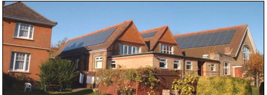
Solar Panels on St Aldhelms Church Hall, Edmonton
